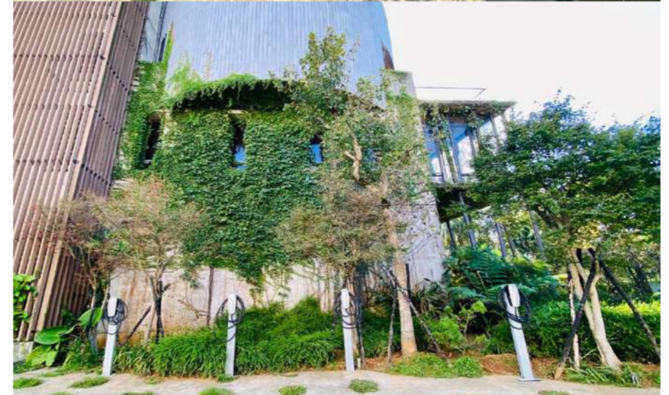
● Figure 1-2 O'right Green Headquarters is the first GMP certified Gold-level green cosmetics plant in Asia and Taiwan's first Diamond-level carbon footprint green building
