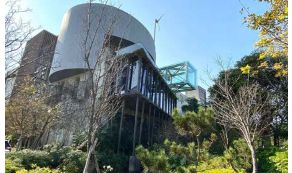
● Figure 1-2 O'right Green Headquarters is the first GMP certified gold-level green cosmetic plant in Asia and the first Diamond-level carbon footprint green building in Taiwan.
